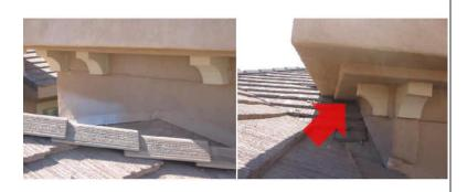
The stucco siding was serviceable, with hairline cracks noted, with exceptions noted.
